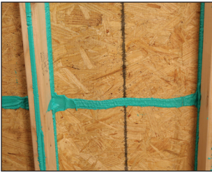
Sheathing Seam Seal
