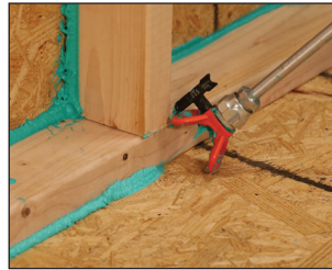
Base Plate to Subfloor Seal
